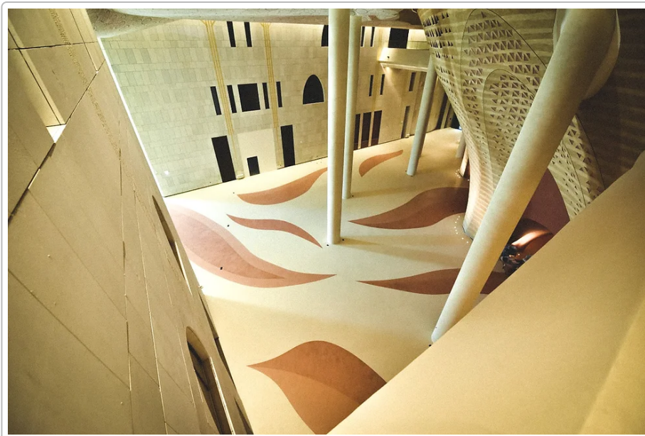
At King Fahad Cultural Center in Riyadh, over 9,000 m 2 of Microdur Plus microcement flooring was installed across high-traffic public areas. The seamless floor design, shown above, incorporates subtle color patterns in a single
