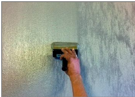
Step 5 - If desired, after a few hours, on a dry wall, apply a second coat to make the effect more full and homogeneous, keeping the vertical direction of the application and drawing FilidiSeta on the wall
