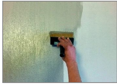
Step 4 - Distribute vertically the product on the wall, to maintain and draw the thready effect of FilidiSeta
